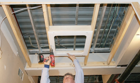
2. Mount Seamless™ surround with drywall with screws
