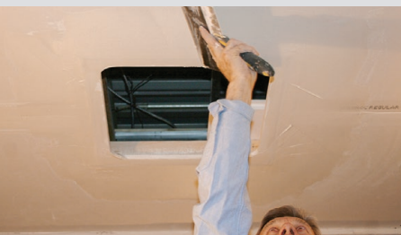
5. Tape and apply drywall compound
