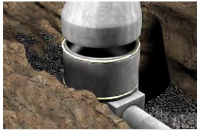
Sealing concrete manhole rings
